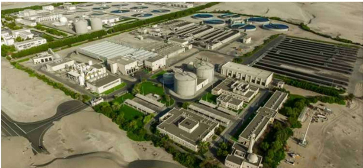
IMAGE 8.1 Al Wathbah-2 WWTP. SOURCE: ADSSC.
