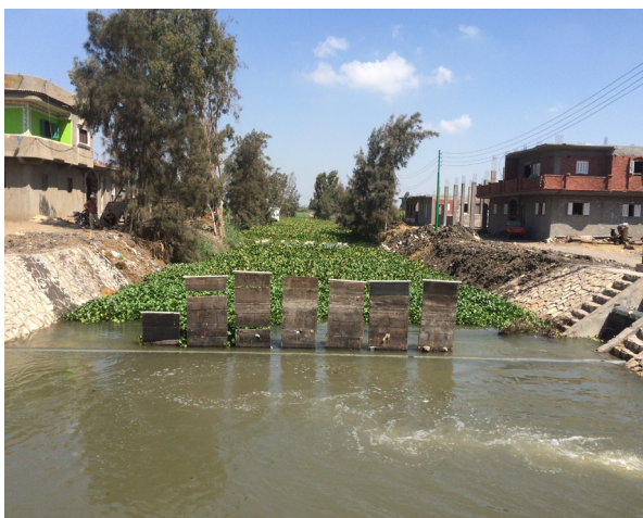
Figure 2: Decentralized wastewater treatment combined with in-stream wetland for reuse in irrigation in rural areas.
